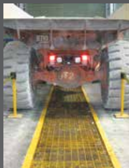
"Wet" pit with grated platform
