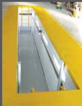
Newly commissioned pit
